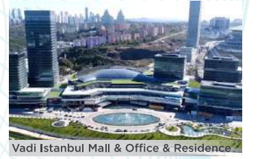
Vadi Istanbul Mall & Office & Residence
